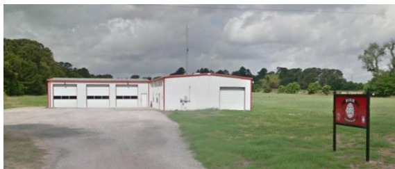
Figure 124: Dixie VFD, Station 2
